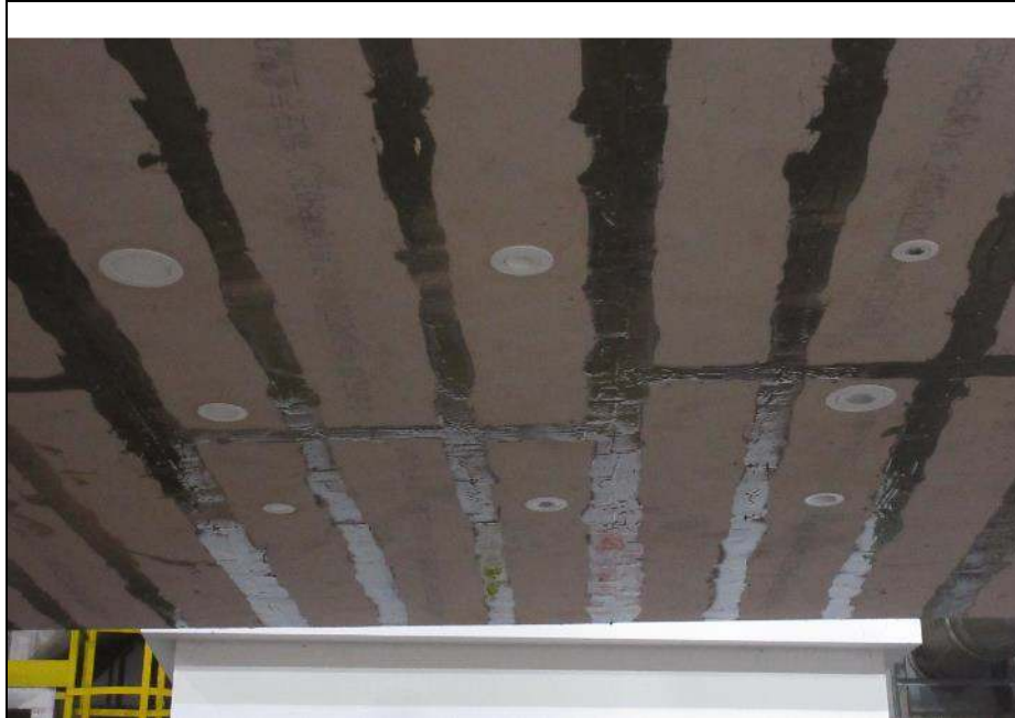
The exposed face before the test
